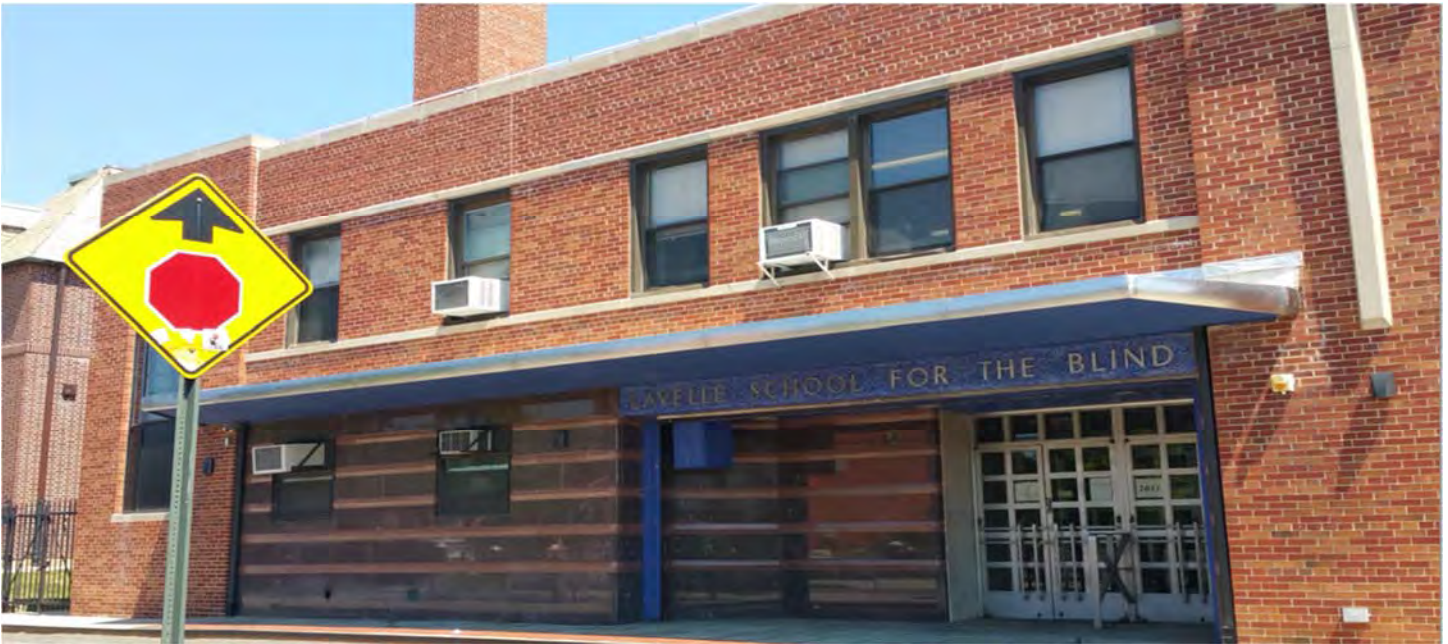
Nearby School for the Blind
